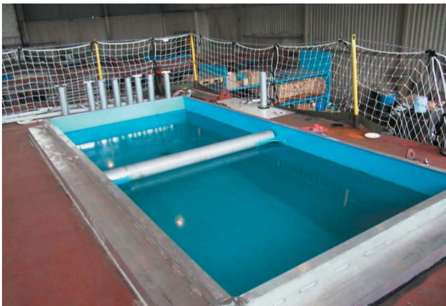
Fig. 1: Adhesive bonded swimming pool.
