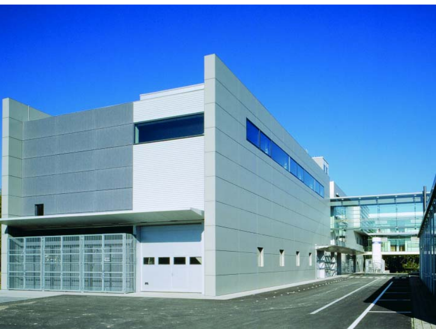
Fig. 1: South side of the foundry hall in Bremen.
