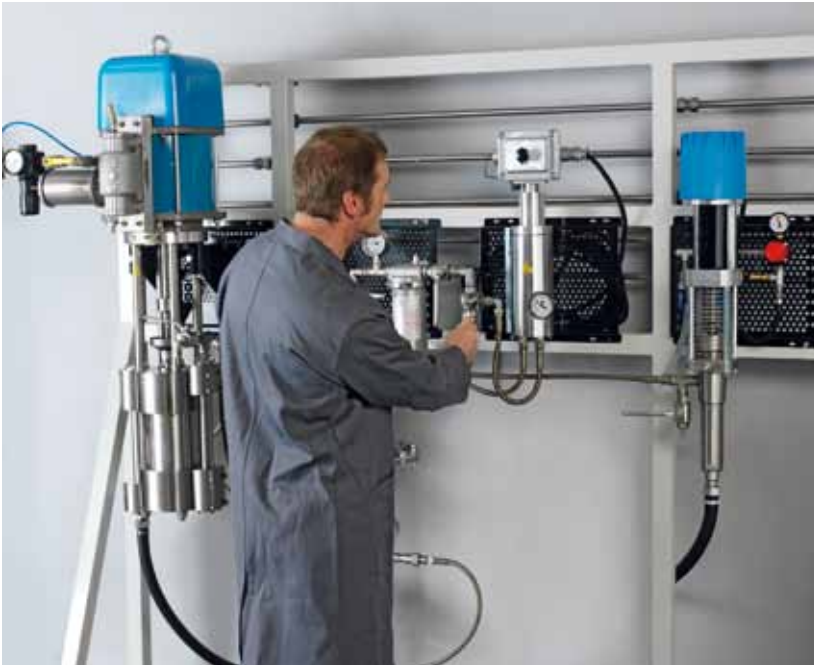
Fig. 1: Test loop at the Fraunhofer IFAM.
